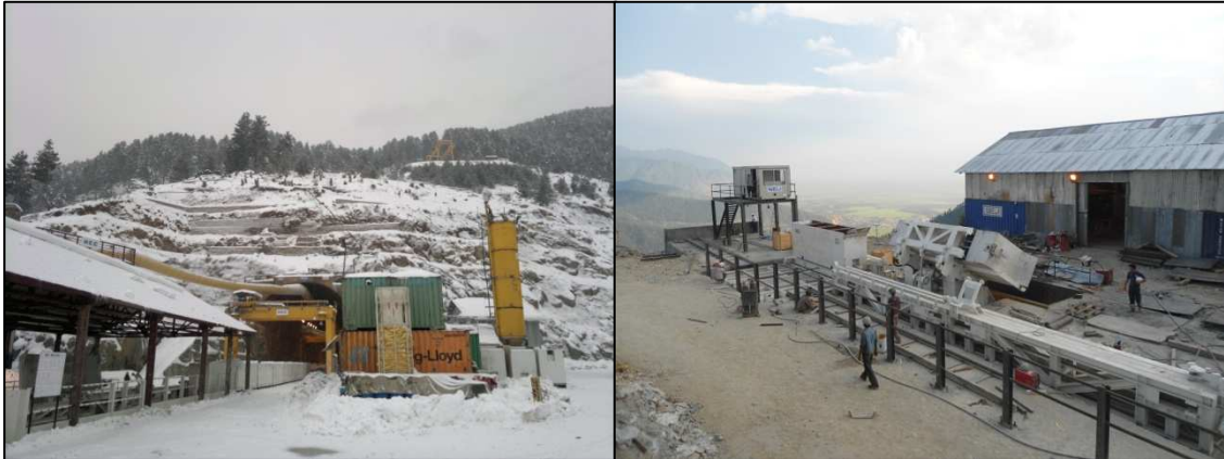
Figures 6. TBM site during winter time (left) and tippler equipment (right)
