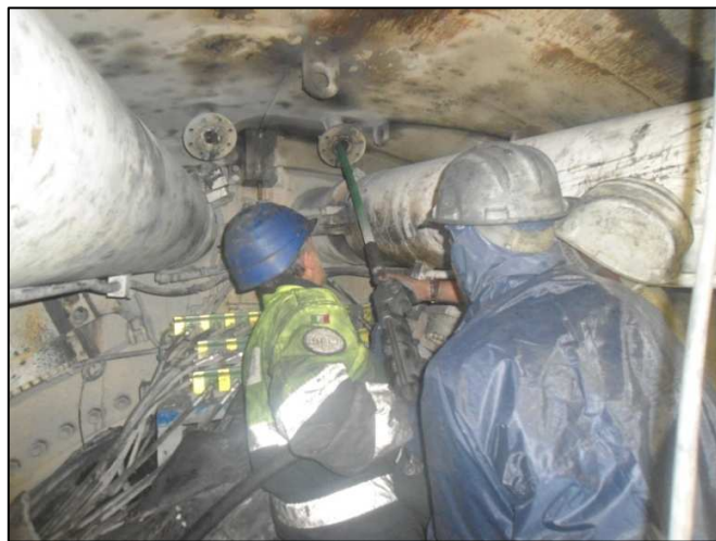
Figure 7. ground treatment at chainage 1+711,87
