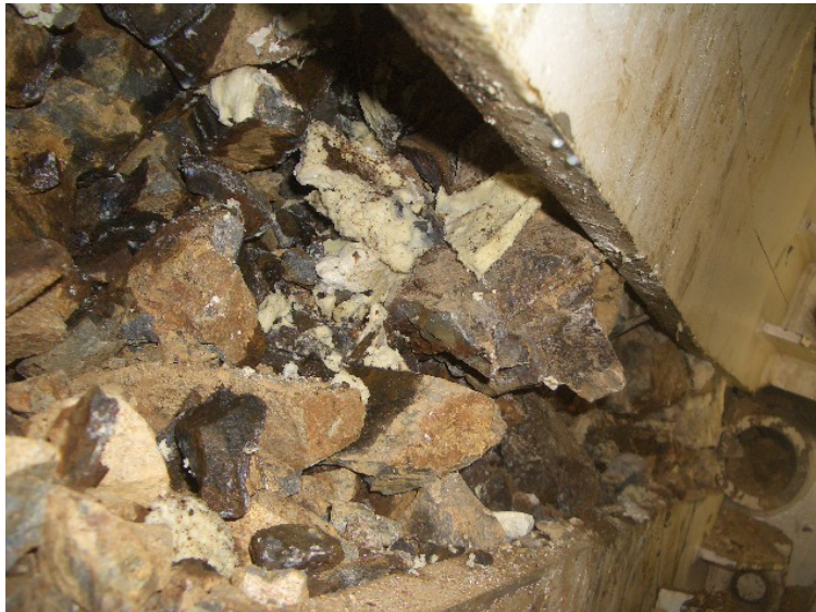
Figure 11. Collapse at the rear shield
