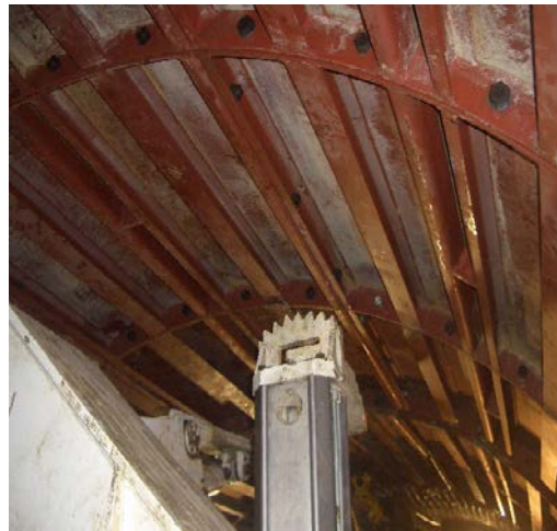
Figure 14. Steel set roof erection
