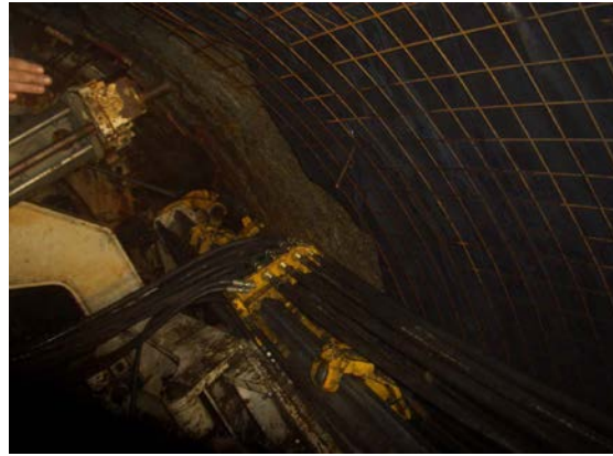
Figure 24. Probe drilling
