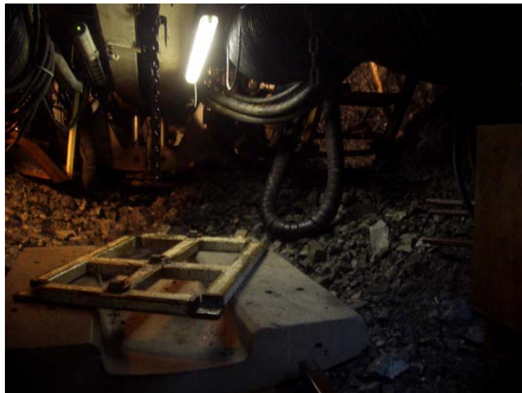
Figure 12. Intruding debris at the invert placing
