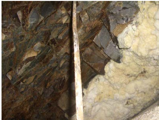
Figure 15. Filling cavity at the front face
