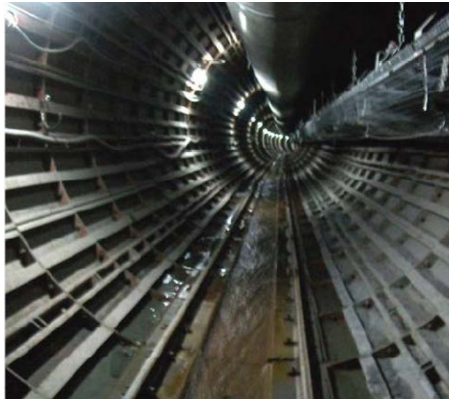
Figure 19. Rock support CS5
