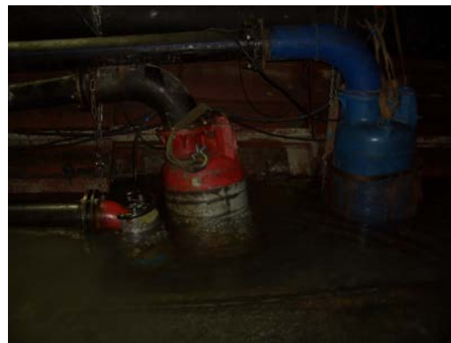
Figure 22. Additional pumping station
