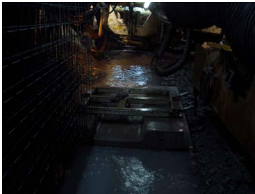
Figure 21. Water and debris at the invert placing
