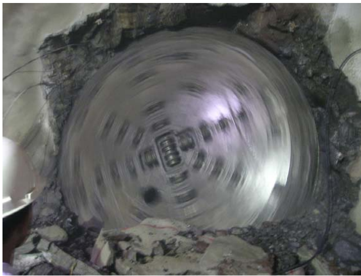
<Figure 14. Breakthrough of the TBM>
