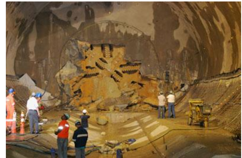
Herrenknecht's EPB shield completes its São Paulo metro tunnel.
